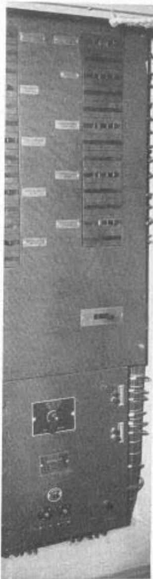
Left—Control locker in coach showing lighting, air-conditioning and radio controls. Right—A regulator locker.
